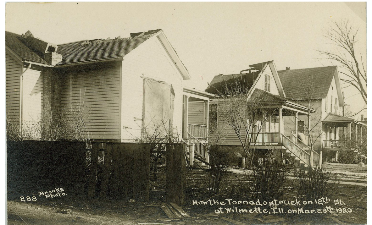
Postcard photo of Wilmette homes damaged in the storm. Photo Courtesy of Frank Suerth
