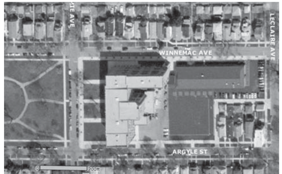
Arial view of the Beaubien School easily shows the additions to the school.
