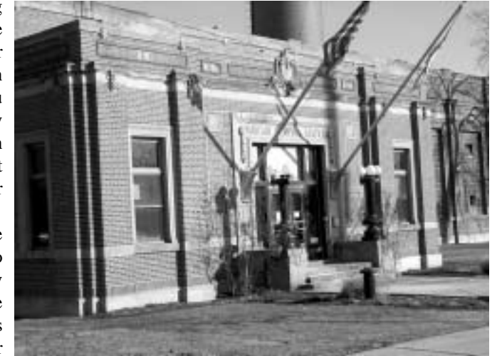
The Mayfair Pumping Station at 4850 W. Wilson
