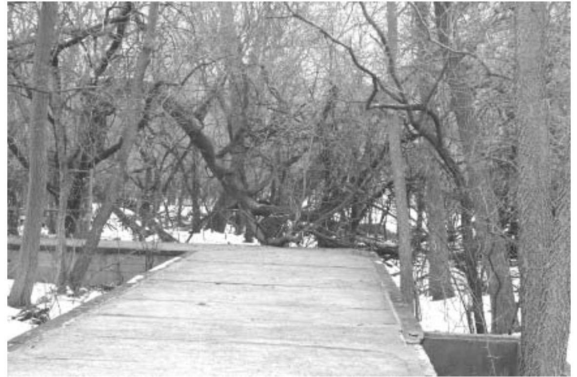
The pavement covers the ceiling of an underground tunnel, part of system that connected all the buildings of the Sanitarium.
