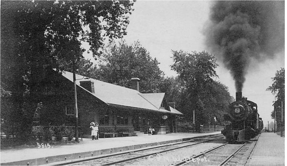
Norwood Park Train Station
