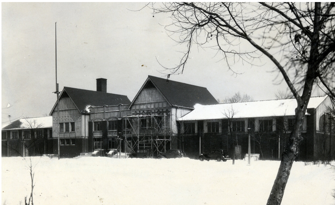
Photo of scaffolding on the fieldhouse at Kosciuszko Park.
