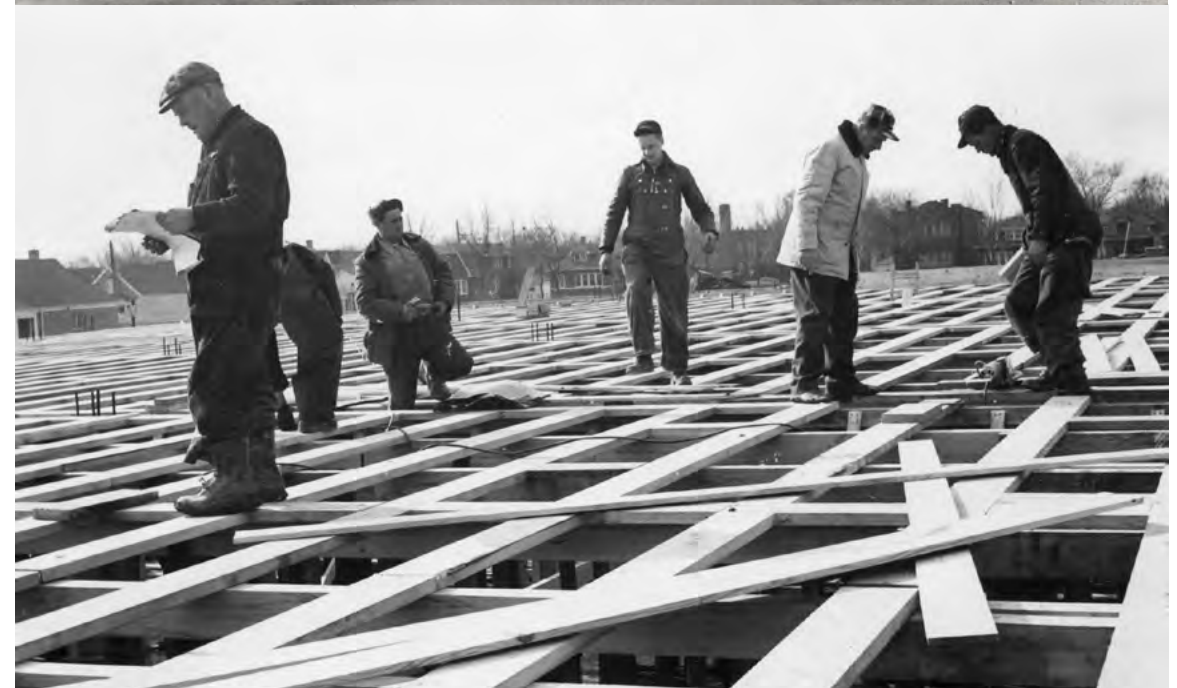
Construction photos for Luther North High School
