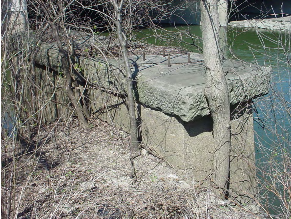
These concrete pylons on each side of the Des Plaines River are all that remains of the Chicago Terminal Transfer Railroad Company's train tracks that ran from Franklin Park to the Mayfair. All other physical evidence has vanished and faded into history.
