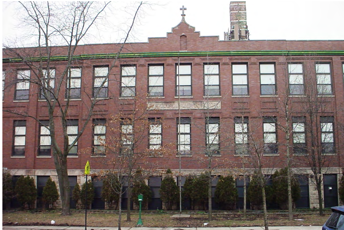
Original School building designed by Herman J. Gaul and was combination, church, school and convent.
