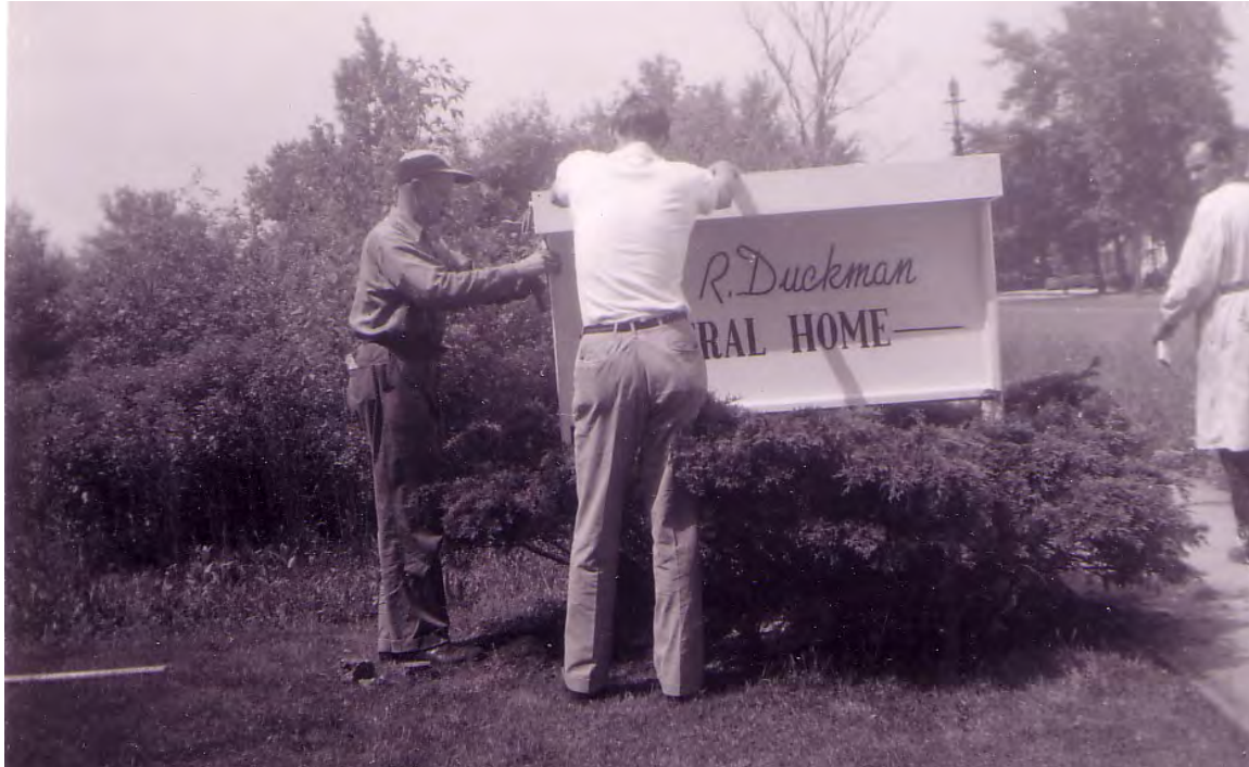
Installing the Fred R. Duckman Funeral sign. Fred is show on the left. Note how rural looking the neighborhood is in the early 1950s.
